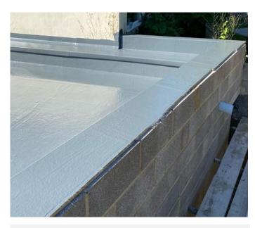
**4/4** A grey resin topcoat (flowcoat) was then applied to the laminate to complete the installation.
