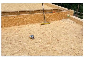
**1/4** BBA® certified OSB3 T&G timber decking installed on the roof. There is BBA® certified PIR insulation sandwiched in between two layers of the decking.
