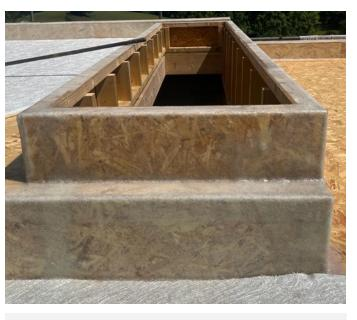
**3/4** Glass fibre matting was applied to the timber decking and saturated in catalysed polyester resin.
