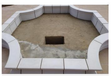
**1/6** Surfaces of the feature were smooth cement screed with any small projections removed to enable the best finish possible.
