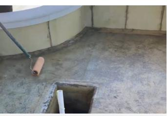
**2/6** Moisture-curing resin primer was applied in a thin layer to act as a barrier to external contaminants and improve laminate adhesion.
