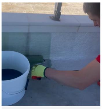
**3/6** Glass fibre matting was applied to the concrete and saturated in catalysed polyester resin using a polyester roller.
