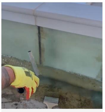
**4/6** The laminate was then consolidated using a paddle roller to ensure good adhesion to the concrete base and a uniform finish.
