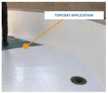
**4/4** A white resin topcoat (flowcoat) was then applied to the laminate to complete the refurbishment.
