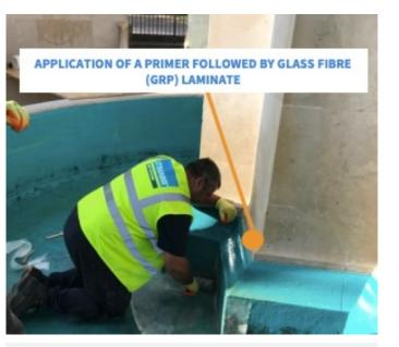
**3/4** Glass fibre matting was applied to the concrete and saturated in catalysed polyester resin.
