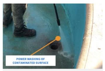
**2/4** Excess dirt and grease were removed via an abrasive method. The surface was then cleaned and dried.
