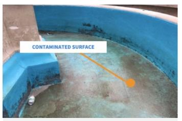
**1/4** Since this was an existing water feature, some additional refurbishment was required prior to laminating.
