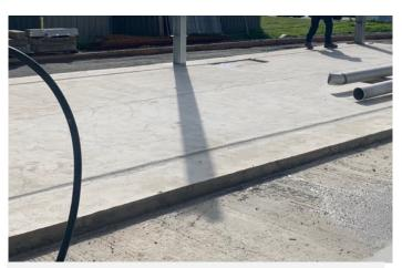
**1/4** Concrete base, uncoated, permeable and porous. This was dried out to remove moisture and excess dust and debris removed.
