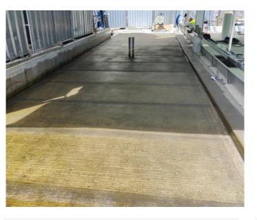
**3/4** A vinyl ester-based resin system was installed onto the primer-coated concrete. A veil was applied on top of the laminate for added reinforcement and chemical resistance.
