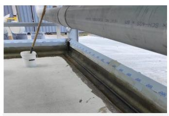
**2/4** A primer was applied to the concrete (in the instance the perimeter drainage systems) to maximise laminate bonding in Step 3.
