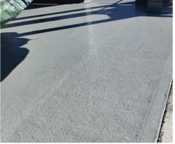
**4/4** A grey, chemically resistant vinyl ester resin topcoat (flowcoat) was then applied with a non-slip finish to the laminate to complete the installation.
