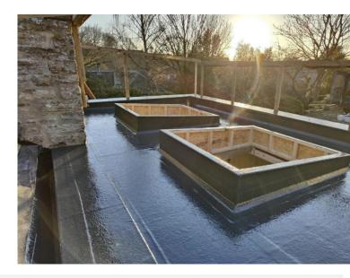
Once the fibreglass laminate had cured, it was mildly sanded back and cleaned prior to the application of a grey flowcoat. This then presented the flat roof amenable to the installation of rooflights.
